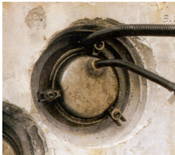
Figure 3.4 Metal Grout Cap 27
