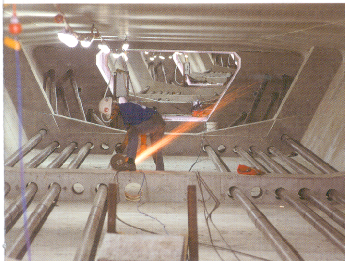
Figure 2.5 Interior of an Externally Post-Tensioned Box Girder 7
